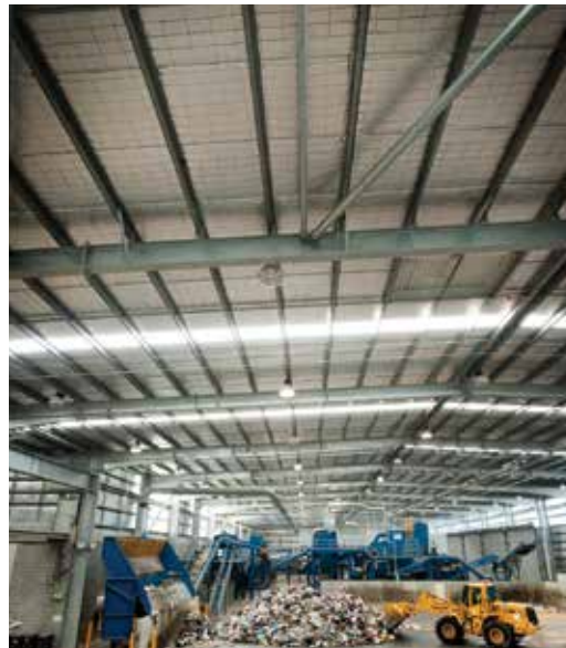
ZAM® roofing purlins at waste recycling centre
